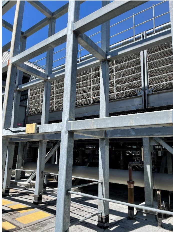
Figure 1.3.2 - Stanley Hall Cooling Towers (1872 tons total): existing cooling towers in Phase 1 that will continue to be used to serve the campus
